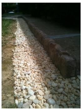
from one or more downspouts. But you must never connect the pipe of an EDS into the same pipe as a buried downspout. In the event of a clog in the line downstream, all of that water would back up into the drain and achieve the exact opposite of it's intended purpose.
